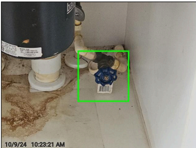
In Kitchen Sink Cabinet
