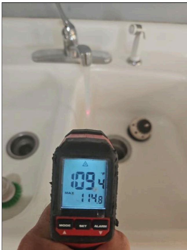
Water Heater Delivering Heated Water
