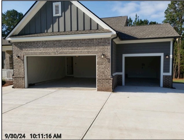
Garage Door and Operator Operational
