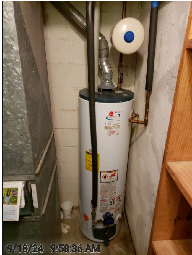
Water Heater and Thermal Expansion Tank
