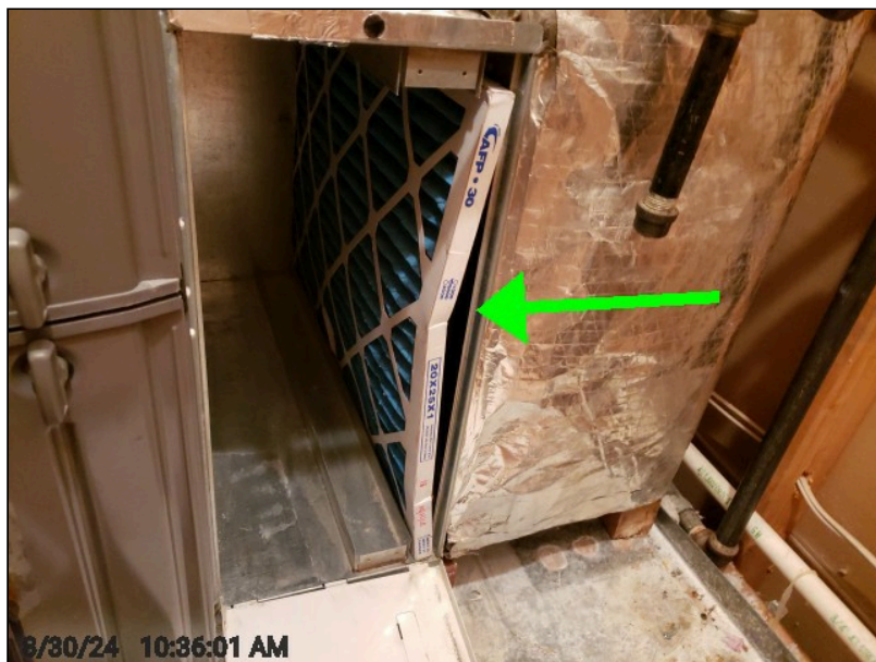
Arrow in the direction of air flow
