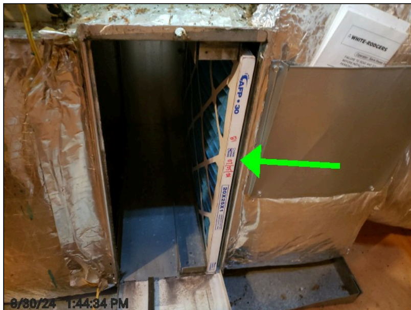
Arrow in the direction of air flow
