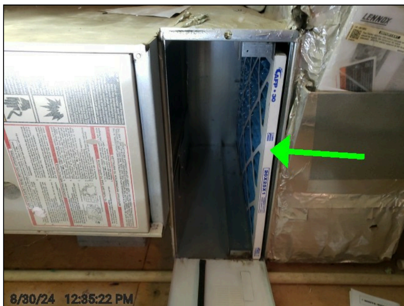
Arrow in the direction of air flow
