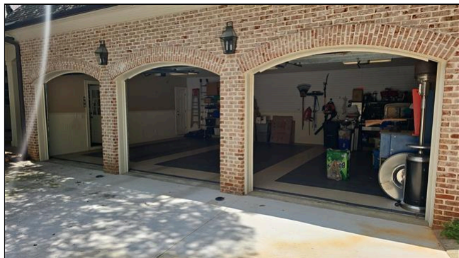
Garage Door and Operator Operational
