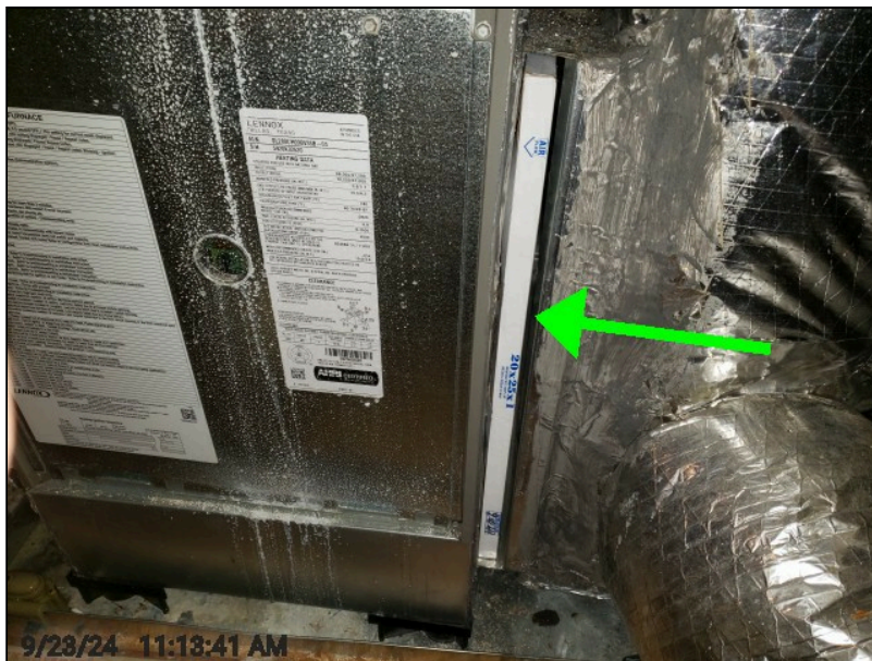
Arrow in the direction of air flow
