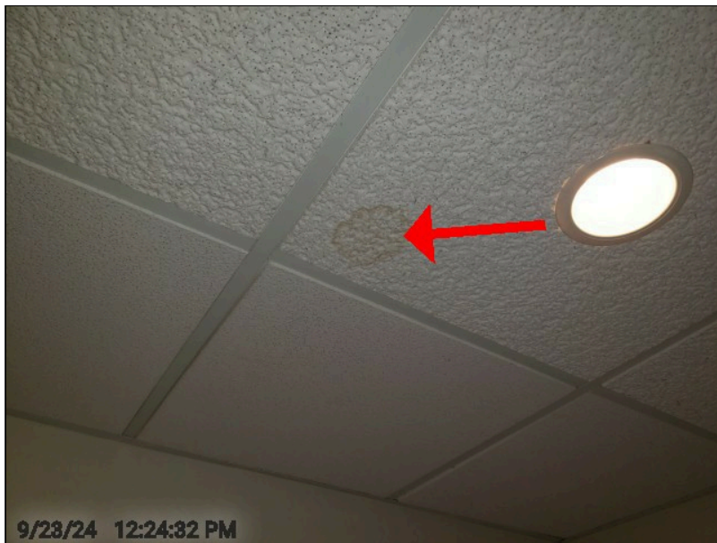
left side of basement
