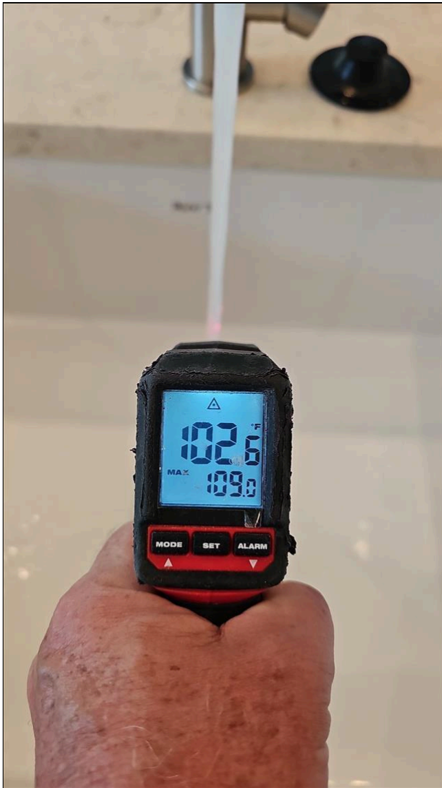
Water Heater Delivering Heated Water
