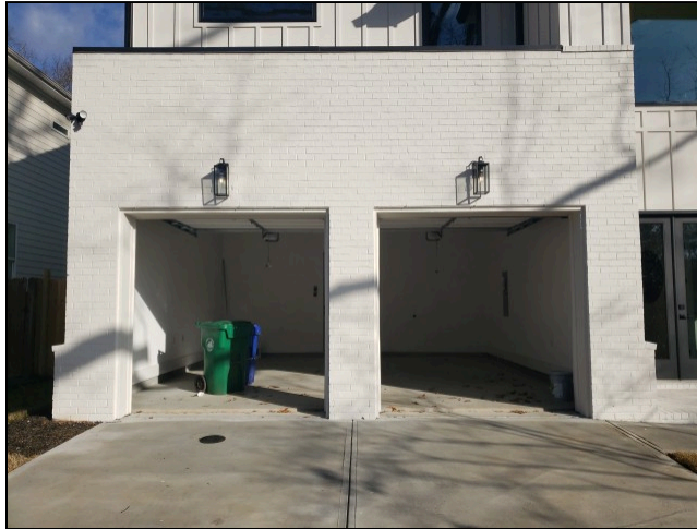
Garage Door and Operator Operational
