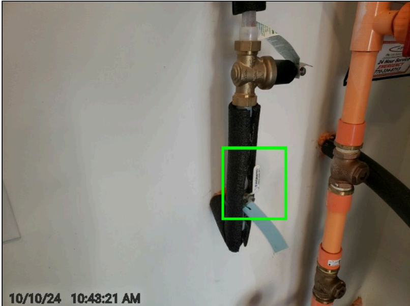
(2) Location of main water cut off to water heater (See Photo).
