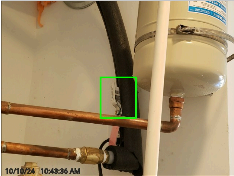
(2) Location of main water cut off to water heater (See Photo).
